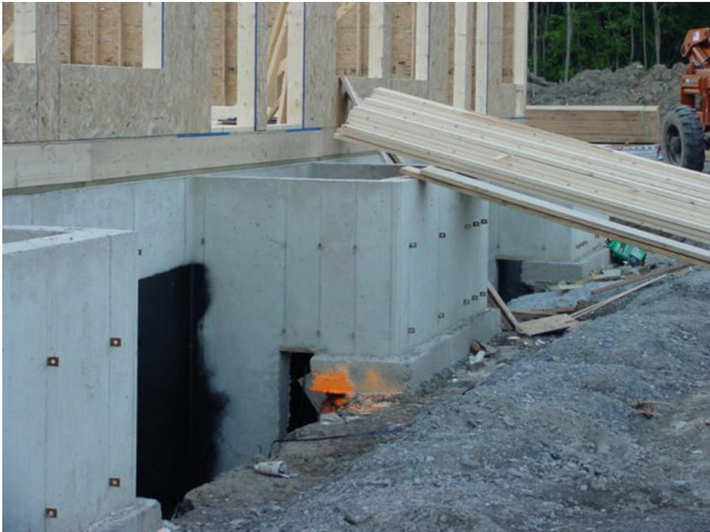
**Photo 14. Erosion of strip footing during construction.**
