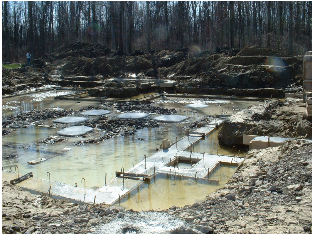
Photo 10. Construction of interior and perimeter footings on stiff stratum in north-central Amherst, NY.
