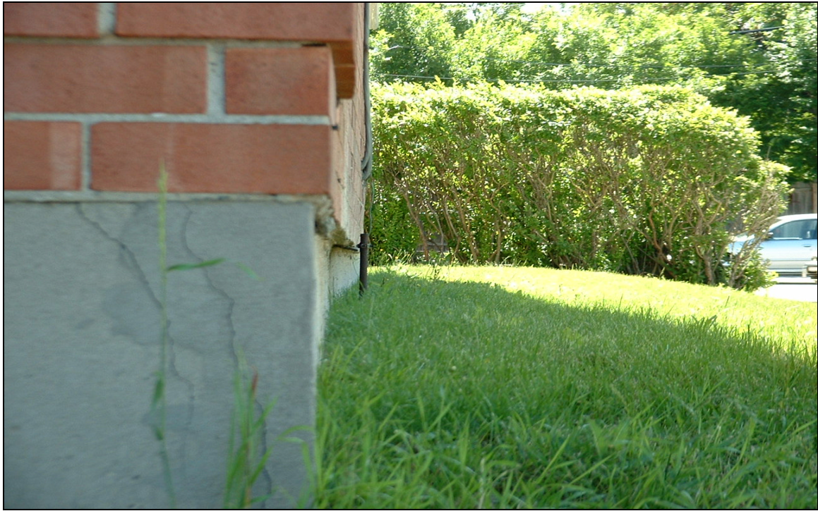
Photo 5. Lateral pressure affecting basement wall in central Amherst, NY. Wall has deflected inward nearly 3 inches from grounding rod.
