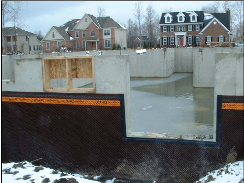
Photo 12. Winter foundation site in East Amherst showing potential for softening from frozen and saturated conditions (March, 2004).
