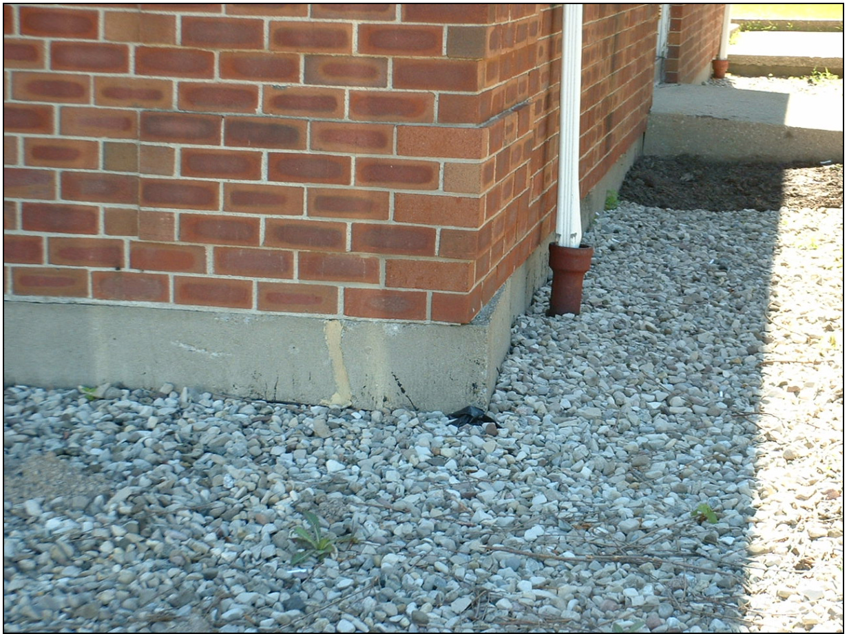
Photo 4. Lateral pressure damage to multi-family apartment complex in south central Amherst (June 2004). Basement walls have corner cracks (patched), and corner block is rotated out. Perimeters soils have settled and pitch into basement wall,; down spouts are often extended and step is settling.
