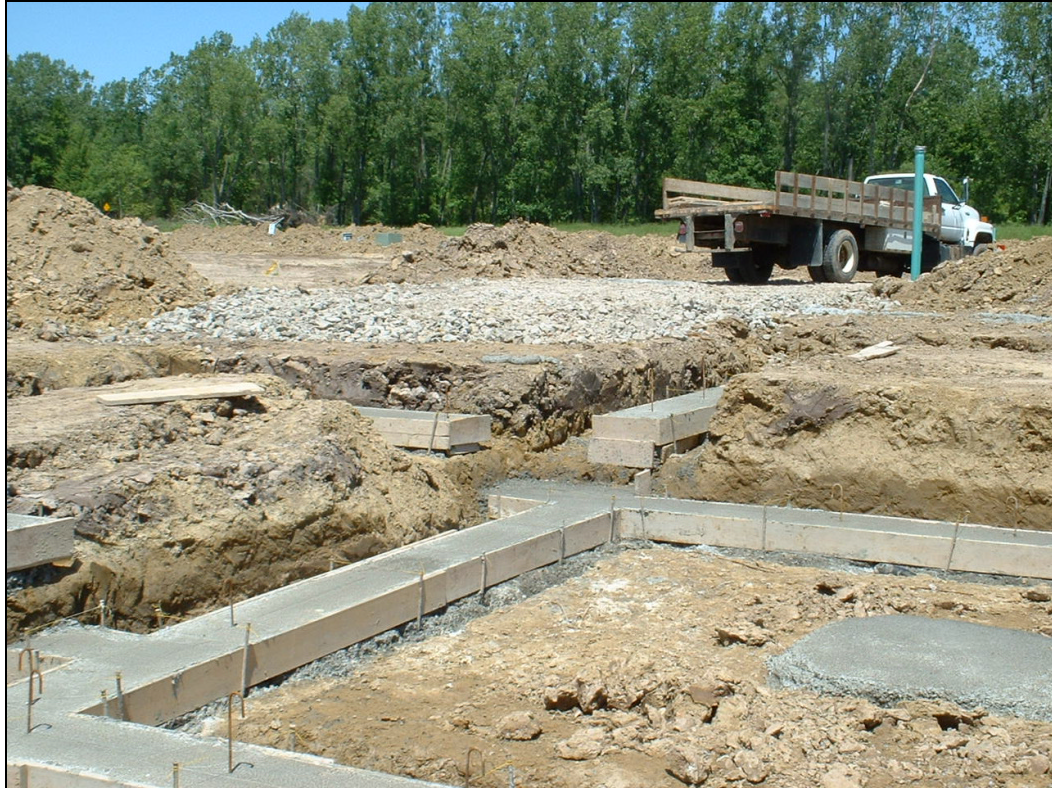
Photo 8. Heterogeneity in shallow soil conditions in north Amherst, NY. Darker soils are clay and lighter brown are fine sand. Note baking of footing soils (c.f., Photo 12).
