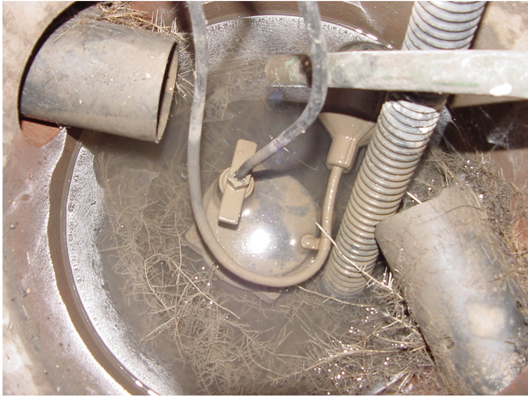
Photo 9. Root hairs penetrating into sump pit in central Amherst, NY.
