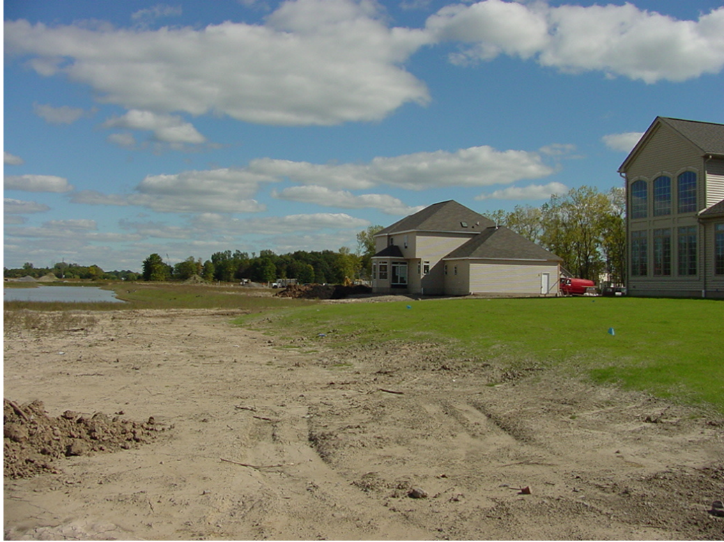
Photo 11. Perimeter loading of house with 3 to 4 feet of fill in northAmherst, NY.
