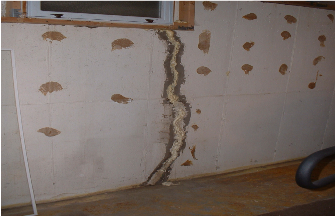
Photo 6. Lateral pressure causing vertical fracture in mid-span of basement wall in north-central Amherst, NY.
