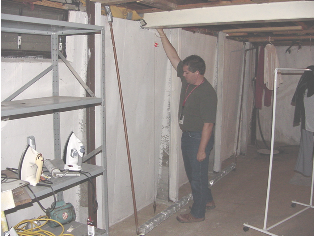
Photo 13. Inward deflection of basement wall (and pilasters) in central Amherst NY. Plum-bob indicates 9" of inward movement. Pipes are damaged and/or relocated.
