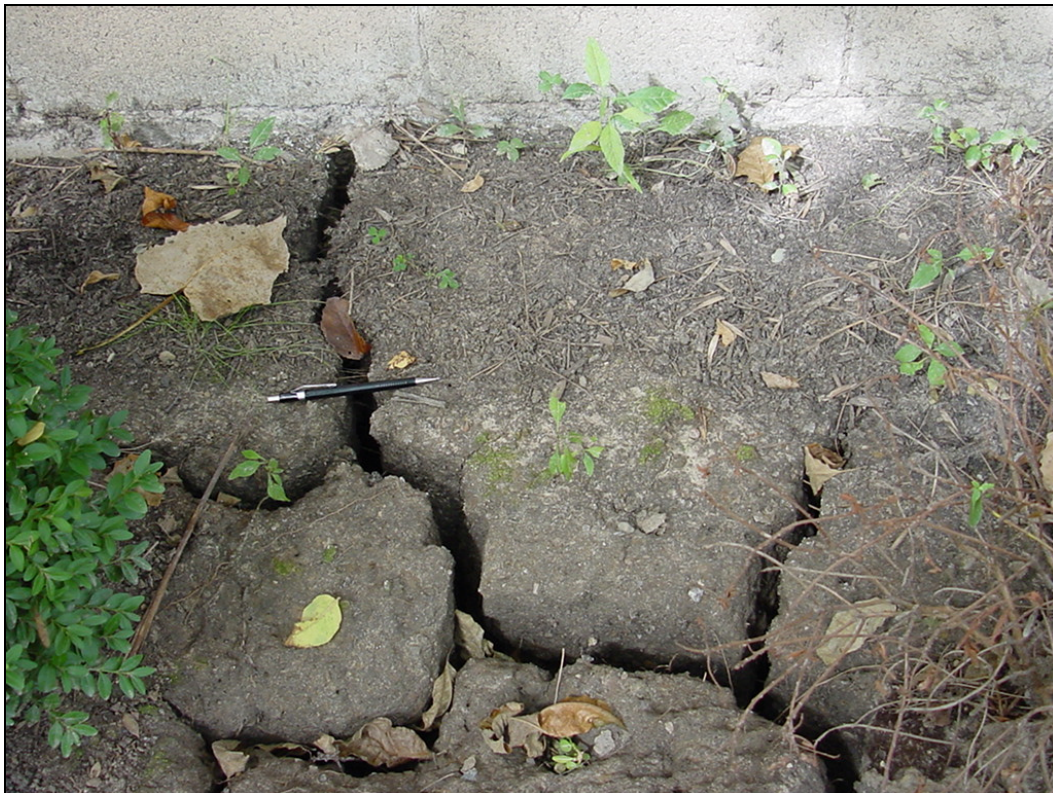
Photo 1. Desiccation cracks in backfill near basement wall in central Amherst, NY, in July 2004.
