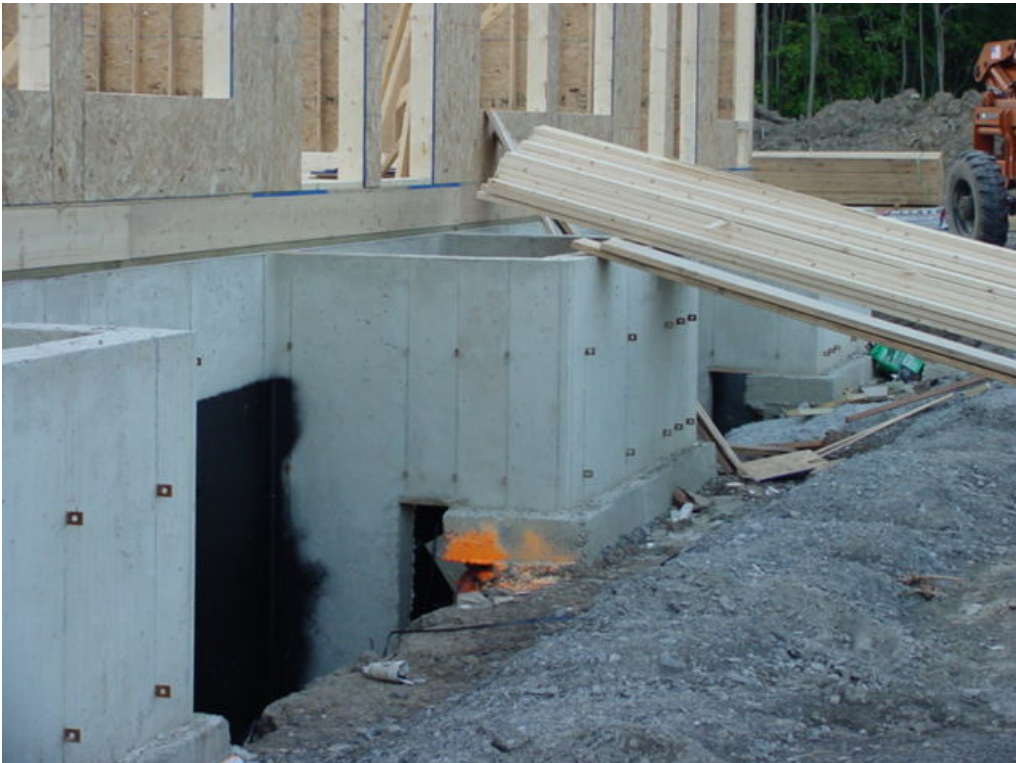
Photo 14. Erosion of strip footing during construction.
