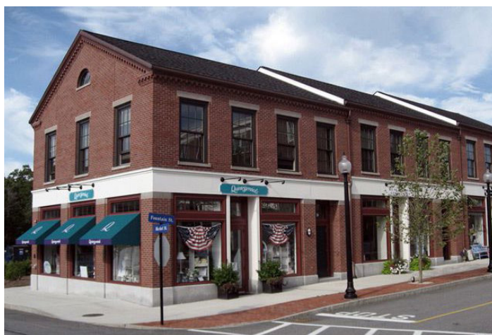
Window trimming in appropriate material, (in addition to other architectural details) helps define the character of a building.
