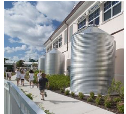
Water recycling systems like cisterns can be exposed (like these) or hidden within the building or site.
