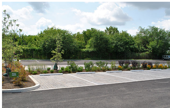
Permeable paving materials and landscaped bioretention areas can help improve stormwater management in parking areas.
