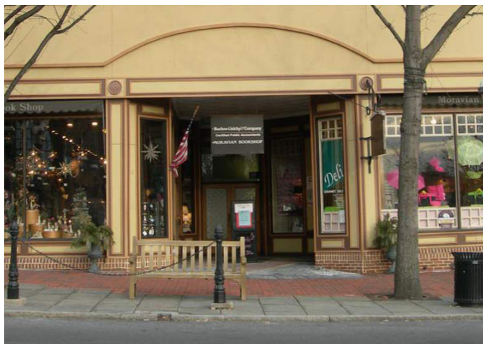
Recessed entries with architectural moldings and other details provide strong visual cues for the location of the main pedestrian entrance on this facade.
