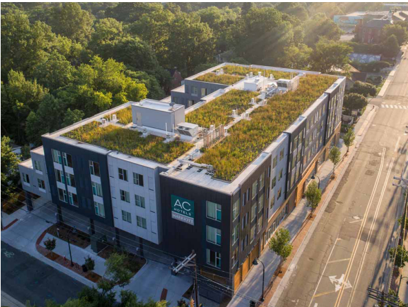
Green roofs help keep buildings and cities cool while providing excellent space for renewable energy production equipment and outdoor amenity space.
