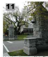
11 Historic gateway on Main Street
