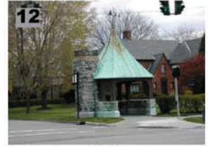
12 Historic gateway on Main Street
