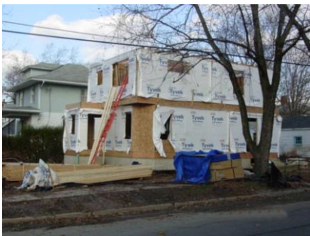
A housing redevelopment project in Eggertsville.
