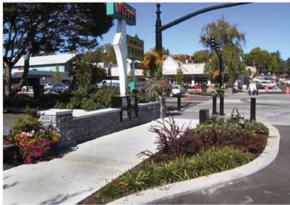
Traffic calming feature (bump out)
