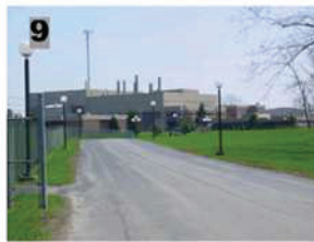
Wastewater Treatment Plant
