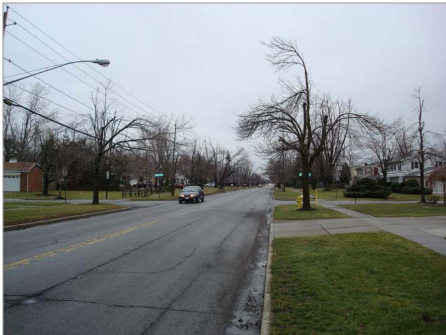
Klein Road looking east from Kingsway Drive
