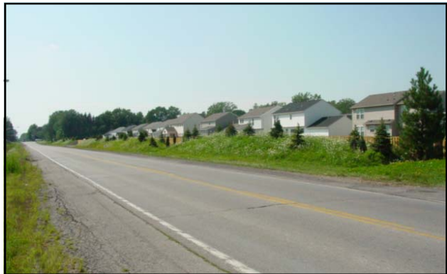
Reverse frontage development along North French Road near Dodge Road minimizes curb cuts.
