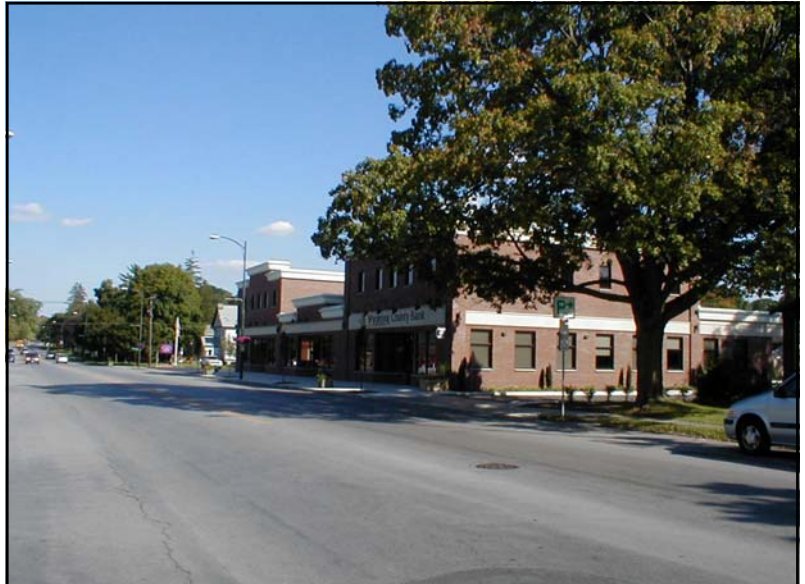
Figure IV-2: Example of new “traditional development” (front view) with on-street parking, zero setback, and appropriate scale to fit with the surrounding development. East Aurora, built 2002.
