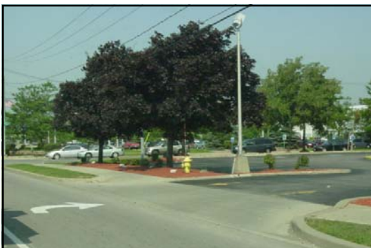
Consideration of driveway consolidation is needed within the functional area of intersections. (East of Bailey Avenue)
