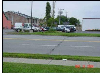
Maple Road east of Old Lyme Road. The existing driveway configuration and drive-thru traffic associated with the business (left photo) coupled with the school traffic across the street (not shown) makes this a difficult intersection to navigate safely. Medians and driveway restrictions could be employed. Future site plan approvals should require additional improvements to internal circulation. Shared access and parking between this business and the adjacent property (right photo) would also improve access.
