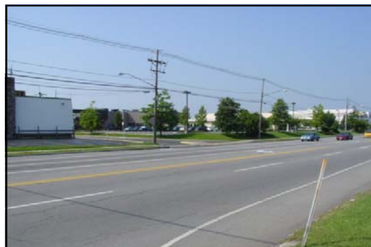
Restricted turning movements to/from directional driveways limit conflict points along Maple Road. (West of Bailey Avenue)
