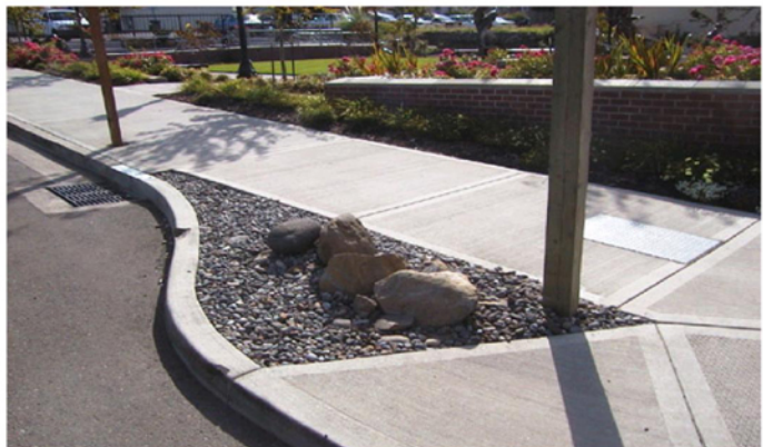
Troutdale, Oregon Bumpout: traffic calming measure
