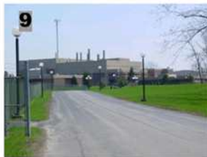
Wastewater Treatment Plant
