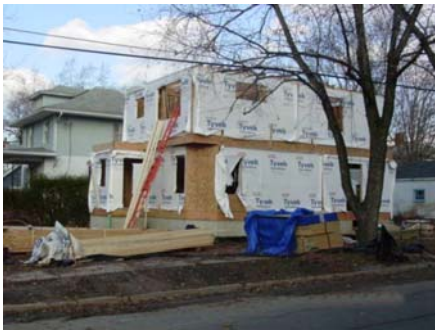
A housing redevelopment project in Eggertsville.
