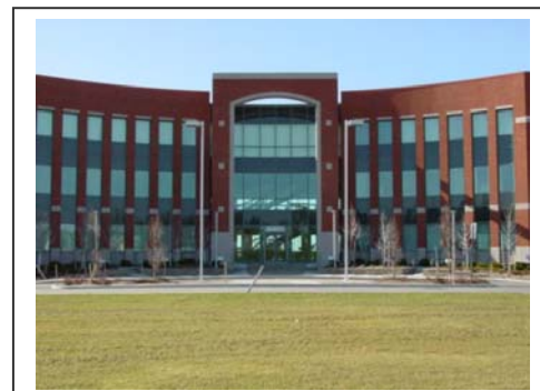
Existing office development at Sheridan Meadows.
