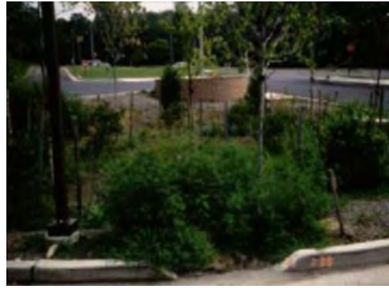
Curb Inlet #2: flow enters through drop curb.
