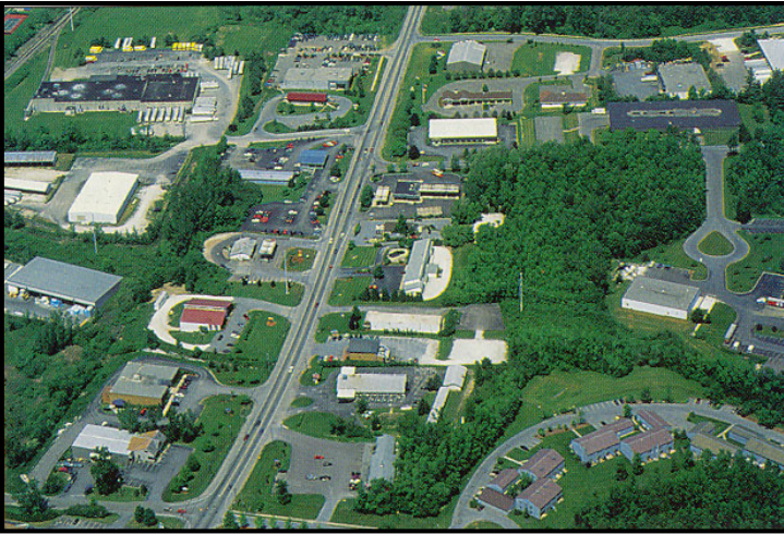
Figure I-5: Typical suburban strip with no access management provisions.
