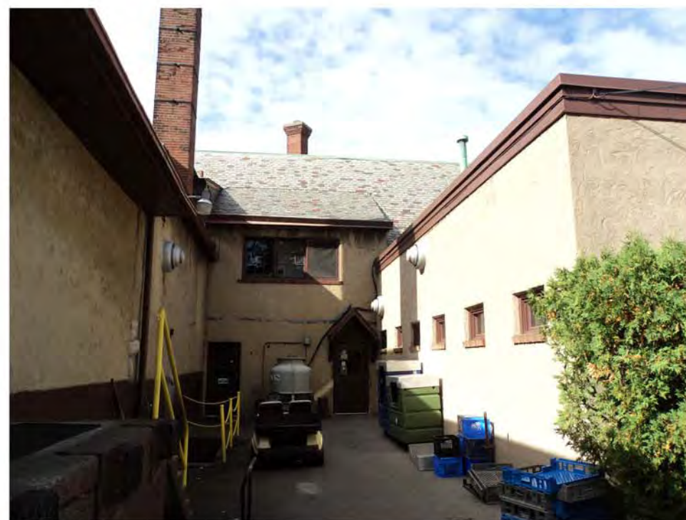
29 Exterior Elevation (Kitchen)
