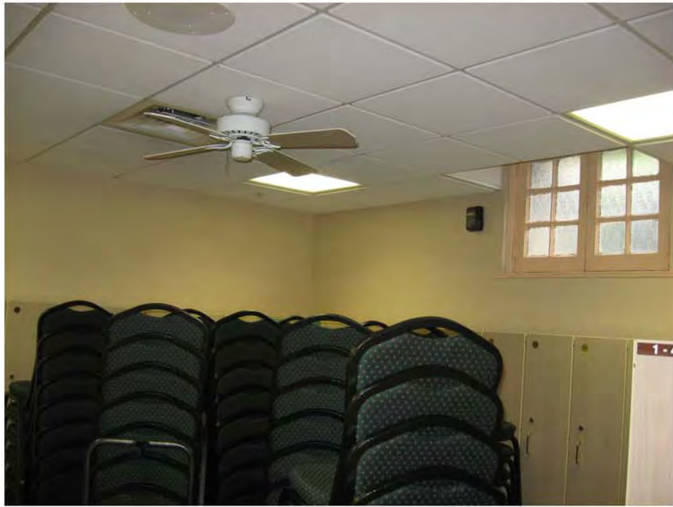
7 Ladies Locker Room
