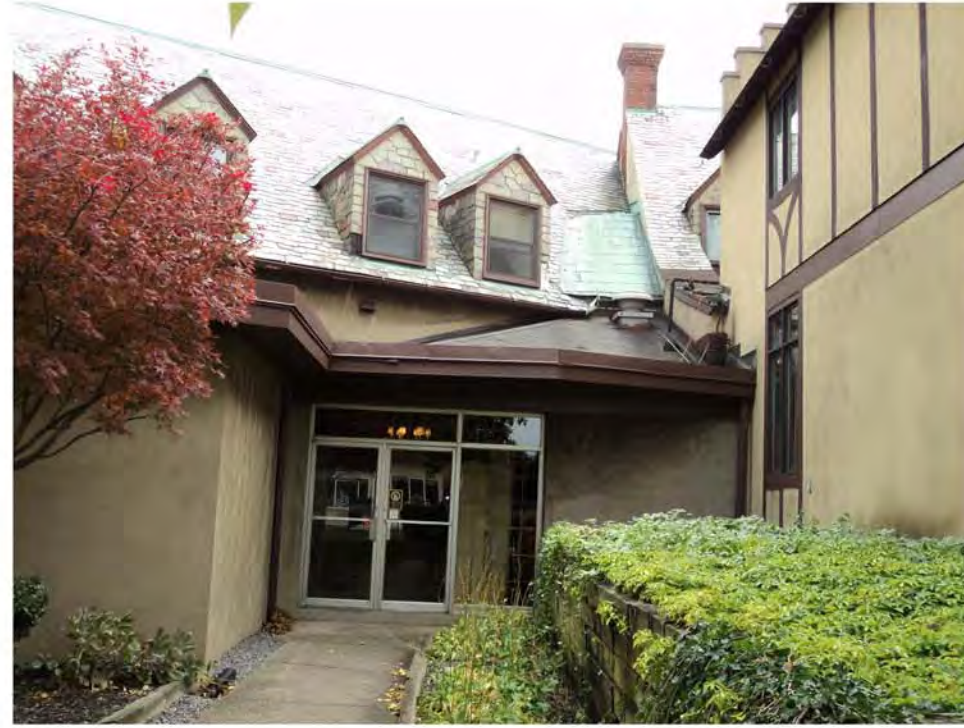
32 Entrance near Bar/Small Banquet Room
