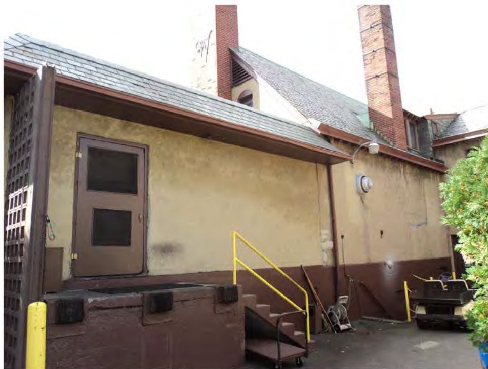
28 Exterior Elevation (Kitchen)
