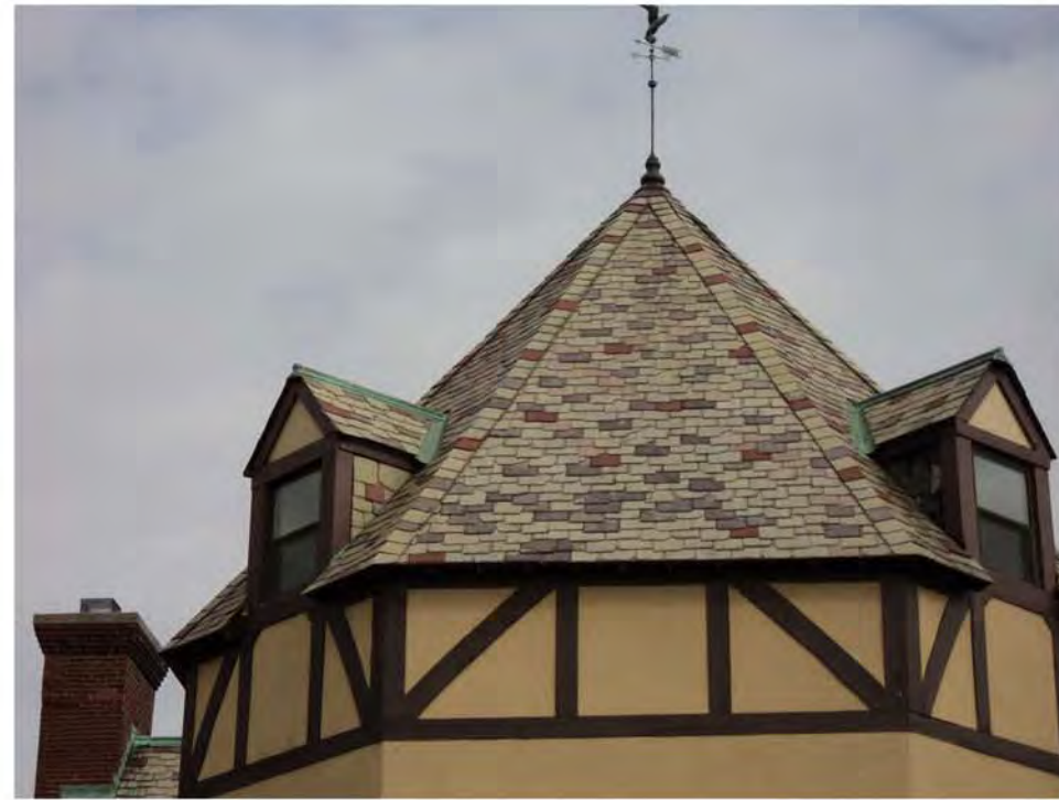
26 Front Entrance Turret
