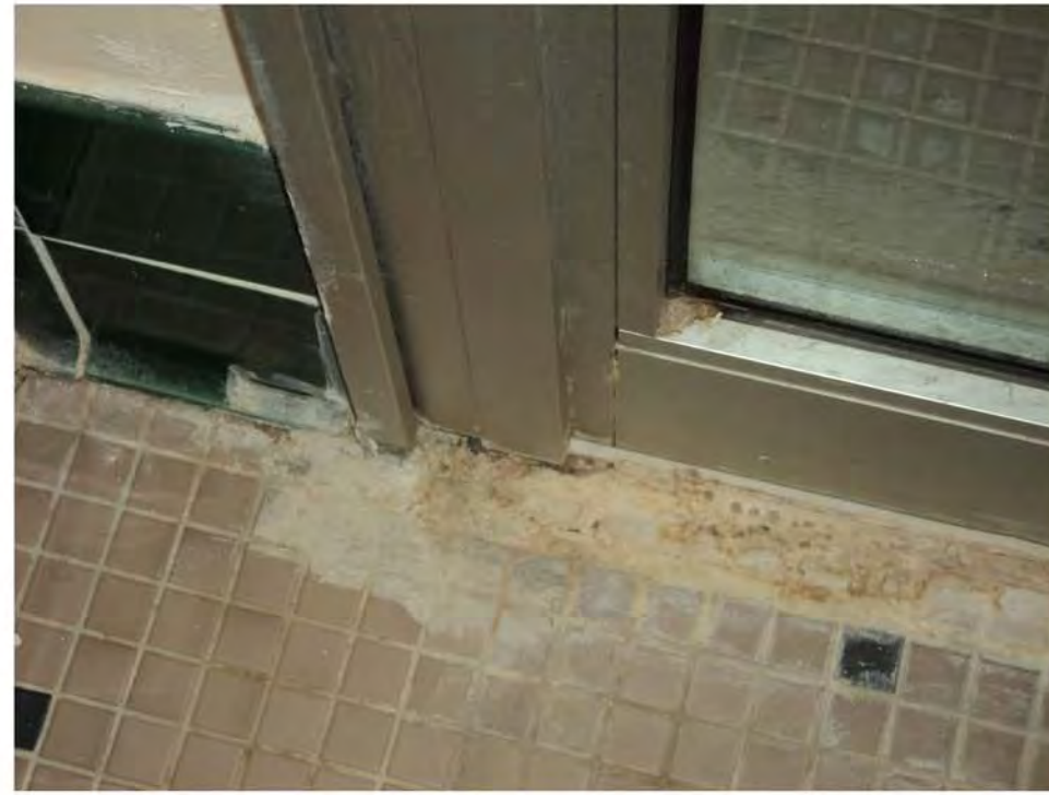
20 Steam Room Entry Door
